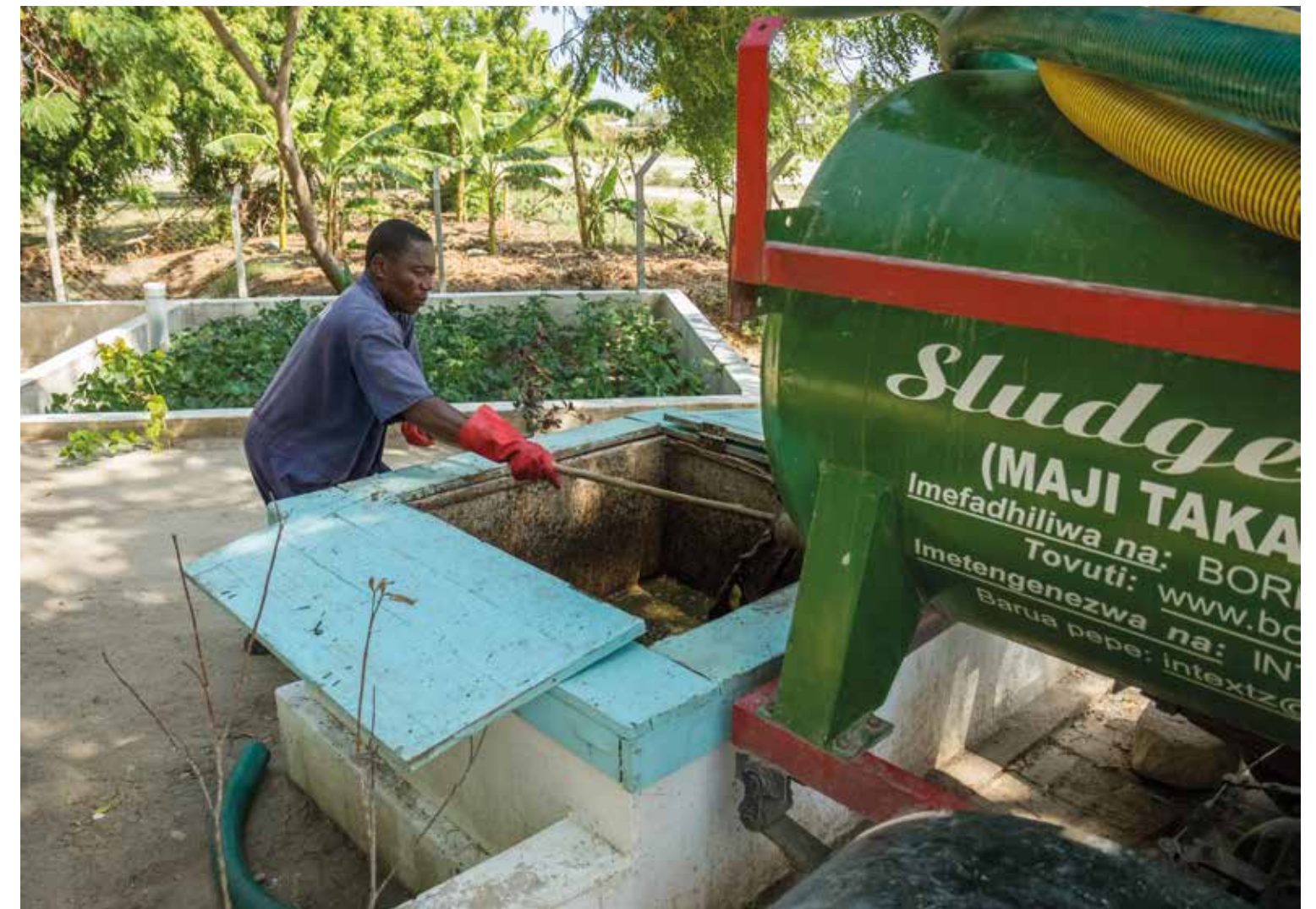
Kigamboni treatment plant →
